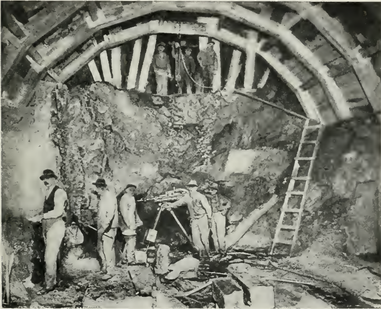
Subway Tunnel Heading at 116th Street and Broadway: Timbering in Soft Ground Over Rock.
